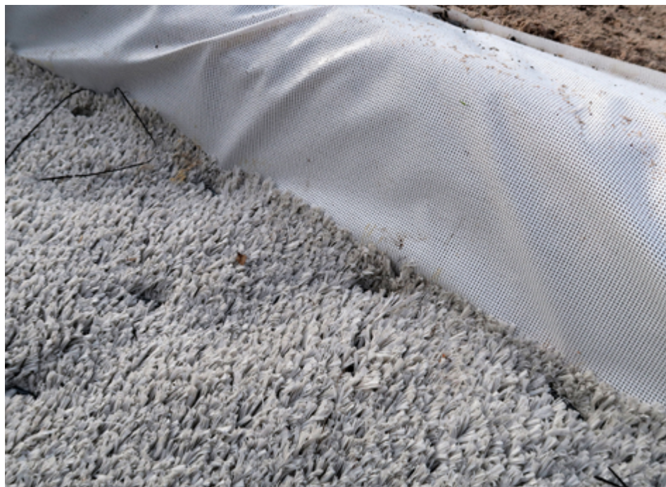
Synthetic turf liners are heavier and more durable than traditional fabric liners. They typically include individual components for the bunker floor, edges, and drain lines.
