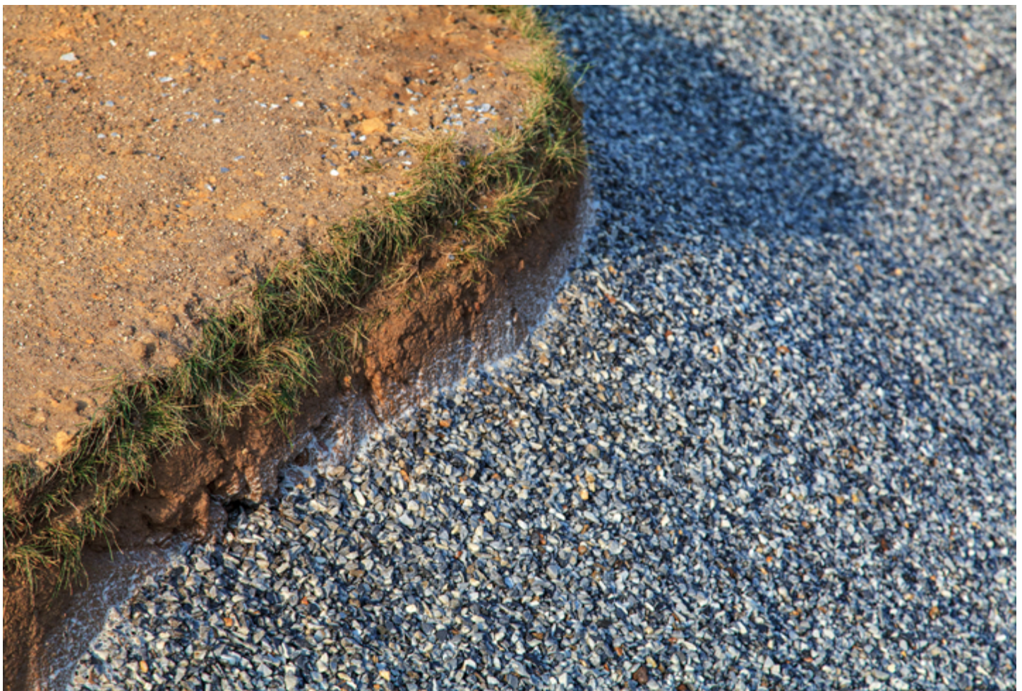
Porous aggregate bunker liners have become increasingly popular for their ability to reduce washouts and sand contamination, but they can be expensive.
