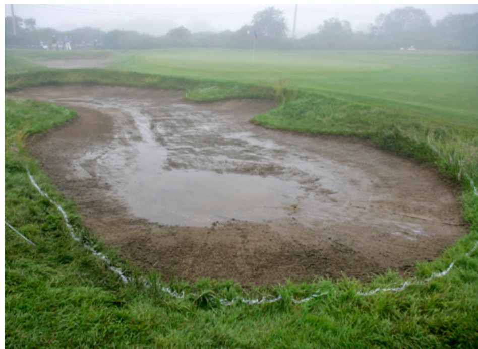
Contaminated sand can leave bunkers flooded and unplayable after a rain event, even if the subsurface drainage system is functioning properly.
