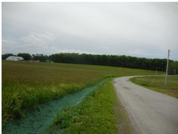
Recently cleaned ditch hydroseeded on Atswell Rd.
