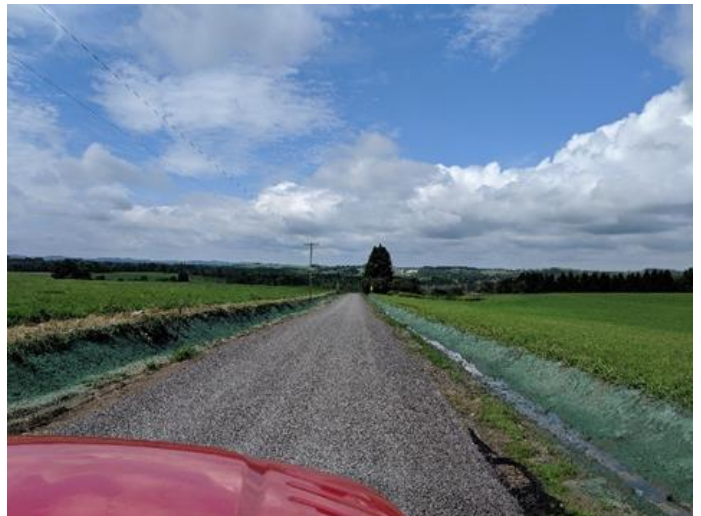
Recently cleaned ditch hydroseeded on Hicks Rd.
