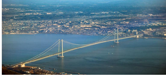
Figure 1. Akashi-Kaikyō Bridge on the Kobe-Awaji Route in Japan
