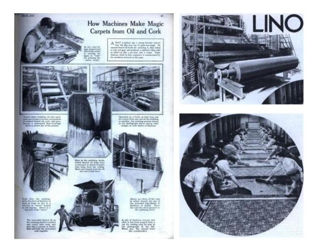
Figure 7: Linoleum Manufacturing Process, Modern Mechanix Magazine, 1922 (left) and 1936 (right), courtesy of Yale
