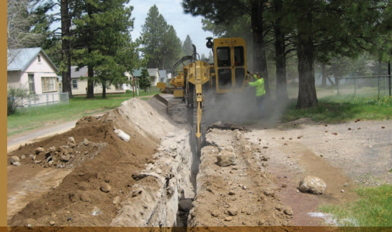
Water line trench
