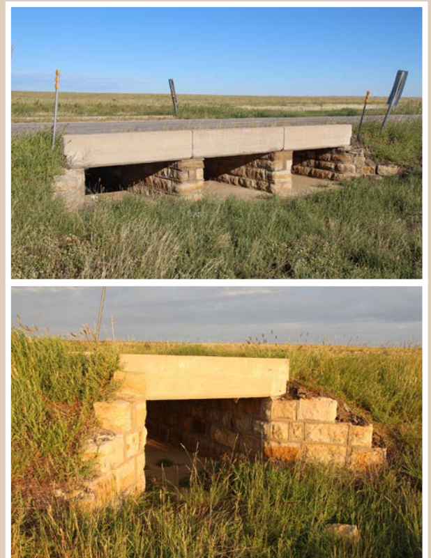
A concentration of four concrete slab bridges and 40 drainage structures built by the WPA along a 20-mile corridor of State Highway 325 in Cimarron County features signs of hand labor, including chiseled masonry substructures (top image – Structure No. 1320 2070 X).
