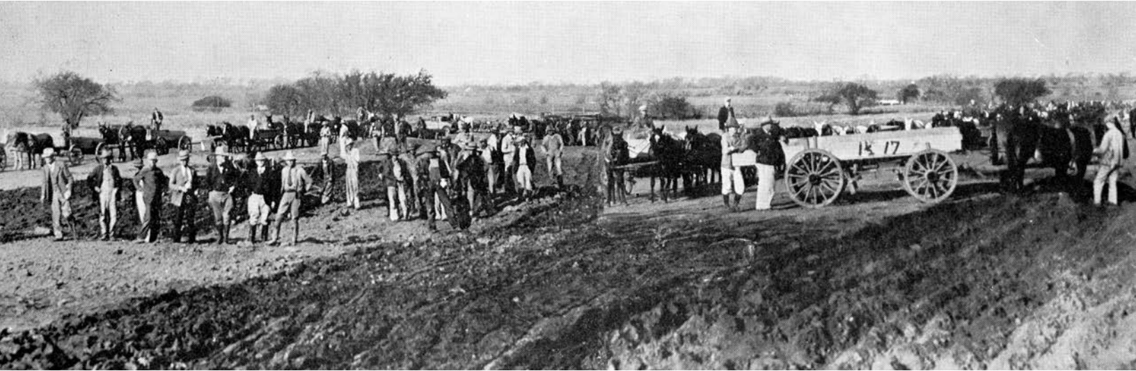
Relief workers surfacing State Highway 36 in Tillman County, 1932.
