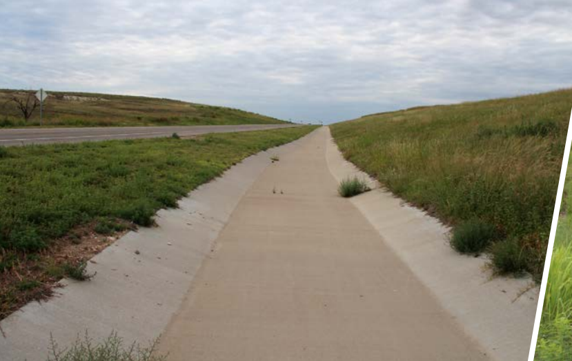
This concrete-lined ditch along U.S. Highway 283 was one of several roadway features financed through a NRWR grant.
