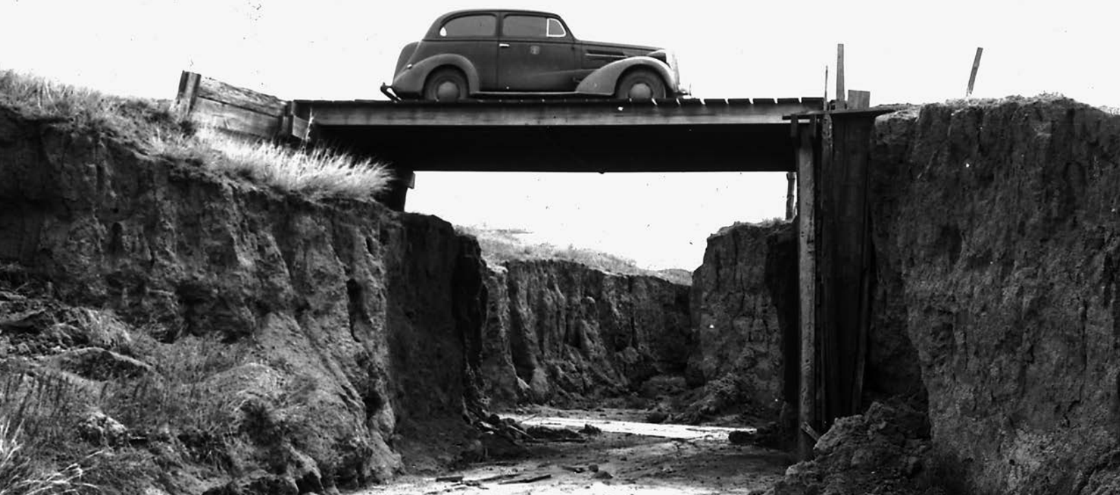
Rudimentary bridges across Oklahoma, such as this one, were in need of improvement or replacement. c.1935.
