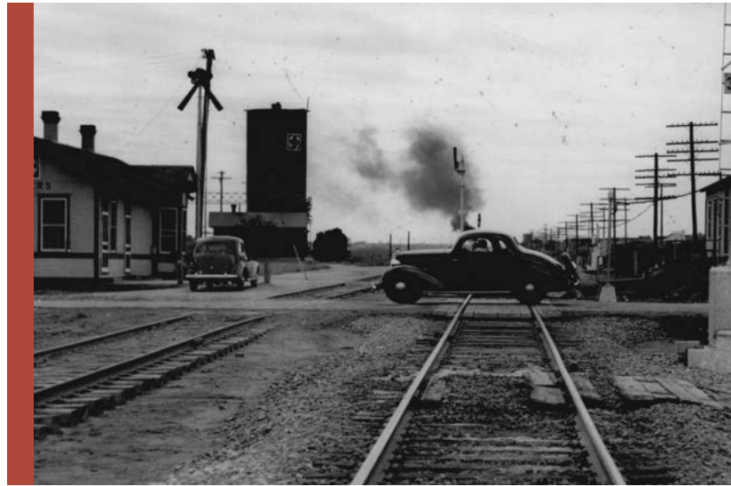
This car crossing a railroad track in 1937 demonstrates dangerous conditions that persisted in many locations across Oklahoma before grade crossings or safety measures were constructed.
