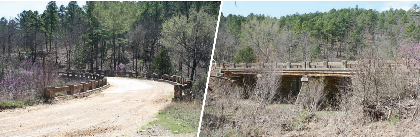
The Rock Creek Bridge is located along a WPA farm-to-market road in Pittsburg County (Structure No. 61N4097E1633000).
