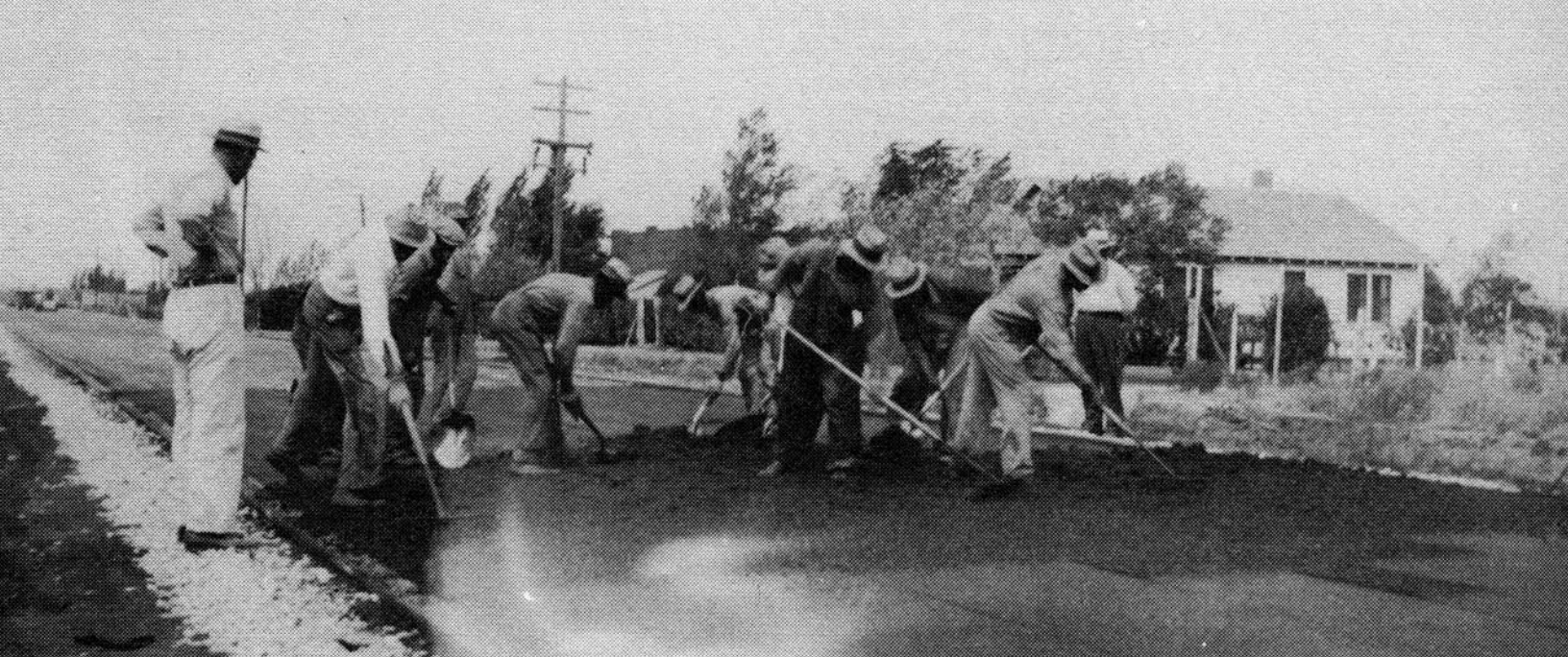
WPA asphalt resurfacing on State Highway 9 in Kiowa County, 1937. This project was completed using hand labor and represents the extensive road-work that the agency undertook throughout Oklahoma.
