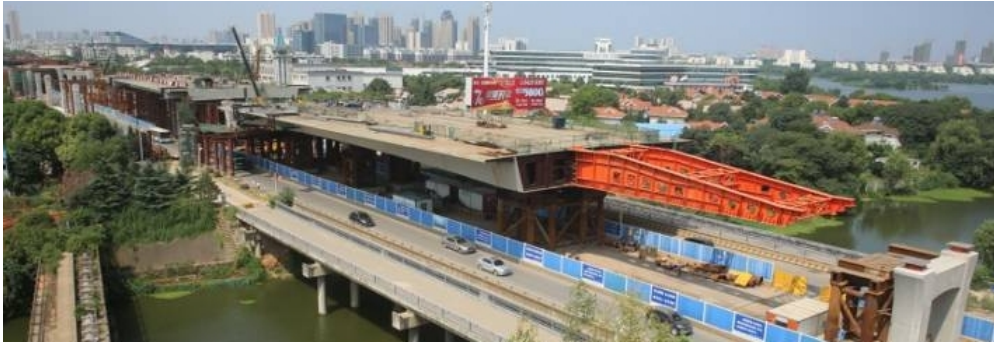
Fig. 5. The launching construction of L7 span of Dongfeng avenue freeway viaduct
