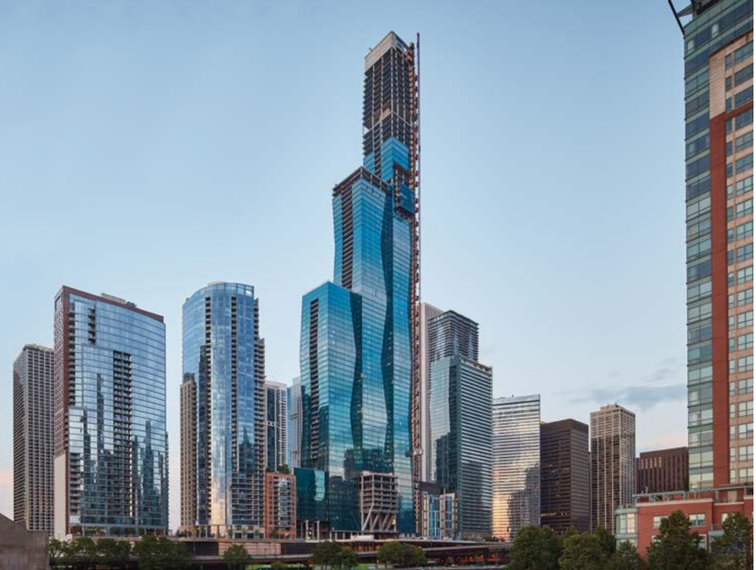
Figure 12. Vista Tower as seen from Lake Shore Drive, showing the blue-green gradient chosen for the final glass application.
