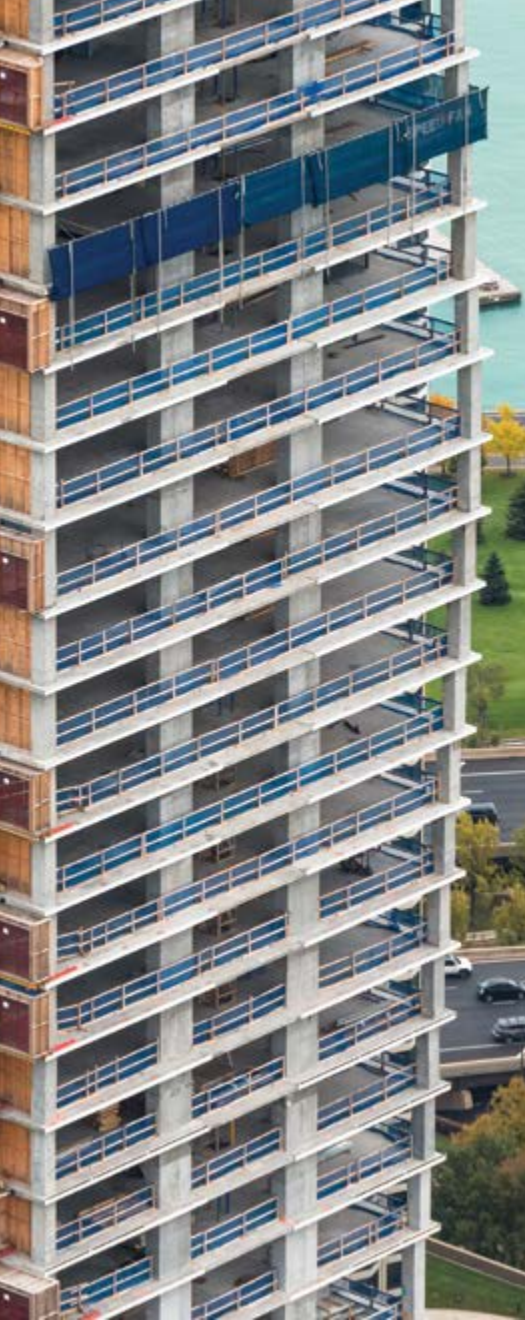
Figure 6. In order to structure the building's stepped edges, "walking columns" align to the outer corners of the floor plates as they step in and out. © Nick Olivieri, courtesy of Magellan Development
