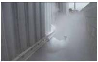
One of the most important aspects when installing ambient vaporizers is to make sure the fog and cold air downdraft being created has the clearance to properly disperse and dissipate to allow new warm air into the vaporizer array. This is done by having the proper clearance from the ground and other surrounding obiects. Walls. tanks. and other vaporizers
