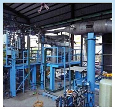
Figure 5 – Microsteam Turbine installed in a Kalina Cycle Power Plant in Taiwan
