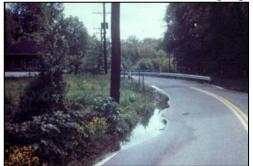
subsurface. Proper surface drainage efficiently removes runoff from the pavement and the nearby ground. Standing water on the pavement or in the side ditches indicates a drainage deficiency. Proper subsurface drainage keeps groundwater from the pavement structure. Two indicators of deficient subsurface drainage are 1) constant water in the side ditch, possibly with cat tails growing, and in the absence of precipitation, or 2) alligator cracking with moisture in the cracks.
