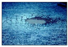
Bowl-shaped holes of varying sizes in the pavement, often resulting from the progressive deterioration of other distresses such as alligator cracking. It usually is caused by a combination of weaknesses in the pavement for the given traffic resulting from insufficient asphalt pavement surface thickness, too many or too few fines, and/or poor drainage. It requires removal of the affected area followed by deep patching with asphalt. *Photo courtesy of the US DOT*.
