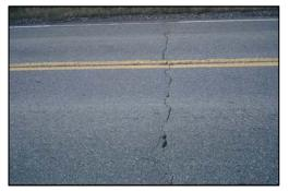
centerline. This frequently is caused by movement in the pavement beneath the asphalt pavement layer (reflection cracking). It can also result from stresses induced by lowtemperature contraction of the pavement. It may require sealing or filling with asphalt material. At a later date, this may be followed by an overlay (eg. tight blade, paver lay) or mill and fill over the entire surface. *Photo courtesy of the US DOT*.
