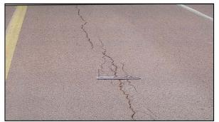
This usually results from a weak joint between paving lanes. These cracks can also result from earth movements, particularly on embankments. Two closely-spaced longitudinal cracks in the wheel path usually indicate bending stress induced by rutting. Longitudinal cracks can also occur as a result of movement in the pavement beneath the asphalt pavement layer (reflection cracking or stripping). For repair, see "Transverse Crack." *Photo courtesy of the US DOT*.
