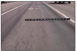
length of at least 20 ft. It is caused by consolidation or lateral movement under traffic in one or more of the underlying courses, or by displacement in the surface layer itself. Ruts should be filled with asphalt (tight-blade) to restore proper cross-section. This should be followed by a thin overlay of asphalt pavement. *Photo courtesy of MnDOT*.
