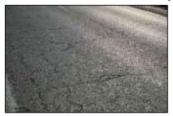
rectangular pieces. Block/multiple cracking is not the result of a structural distress (see alligator cracking), rather it is the result of transverse and longitudinal cracks becoming interconnected. Depending on the severity of the block/multiple crack pattern and dimensions, cracks may be treated by crack sealing, or fog treatment with asphalt material possibly followed by a surface treatment over the entire surface.
