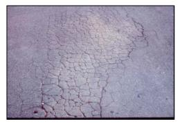
resembles an alligator's skin, and is a load-related structural distress found in the wheel path. It is caused by excessive deflection of the surface over unstable pavement base or subgrade layers that leads to fatigue failure. The unstable support usually is the result of saturated layer or layers or an unstable pavement design. It requires deep patching with asphalt.
