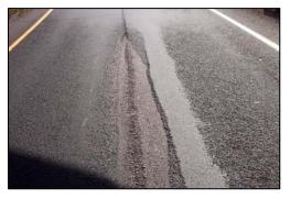
dislodgement of aggregate particles. It is caused by the type, compaction capability original during mix construction, construction during wet or cold weather, or overheating of the asphalt mix. It usually requires a surface treatment of some type. Photo courtesy of MnDOT.
