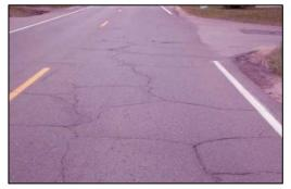
sharp angles at the corners. Shrinkage crack are not related to traffic loading. It is caused by volume change in the base or subgrade. It requires monitoring of the hairline cracks, crack sealing, or fog treatment with asphalt material possibly followed by a surface treatment over the entire surface. *Photo courtesy of MnDOT*.
