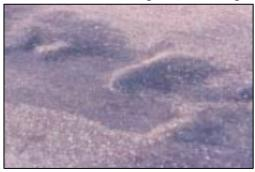
of the surface. It is caused by lack of stability in the subgrade, base, or surface layers. It requires the removal of the affected area followed by deep patching with asphalt. Photo courtesy of FHWA.
