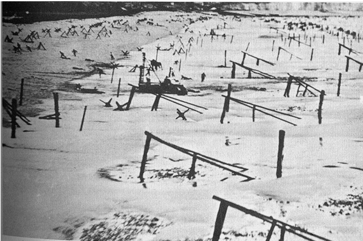
A-3) Ramps, hedgehogs, mine-tipped poles, and tetrahedrons on a Normandy beach.
