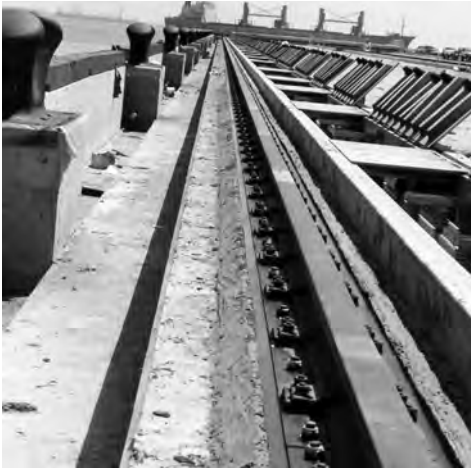
PORTS (CRANE RAILS)
