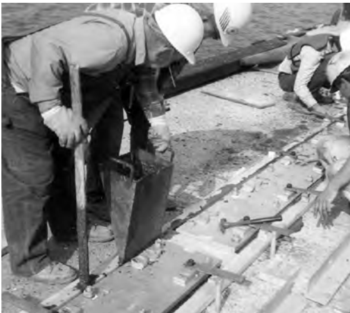
PLUNGING TO ASSIST GROUT FLOW
