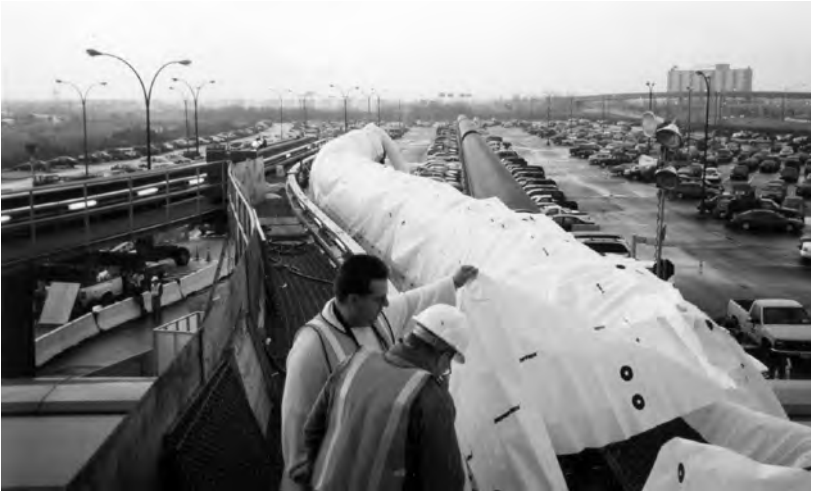
TENTED, HEATED ENCLOSURE FOR COLD WEATHER GROUTING
