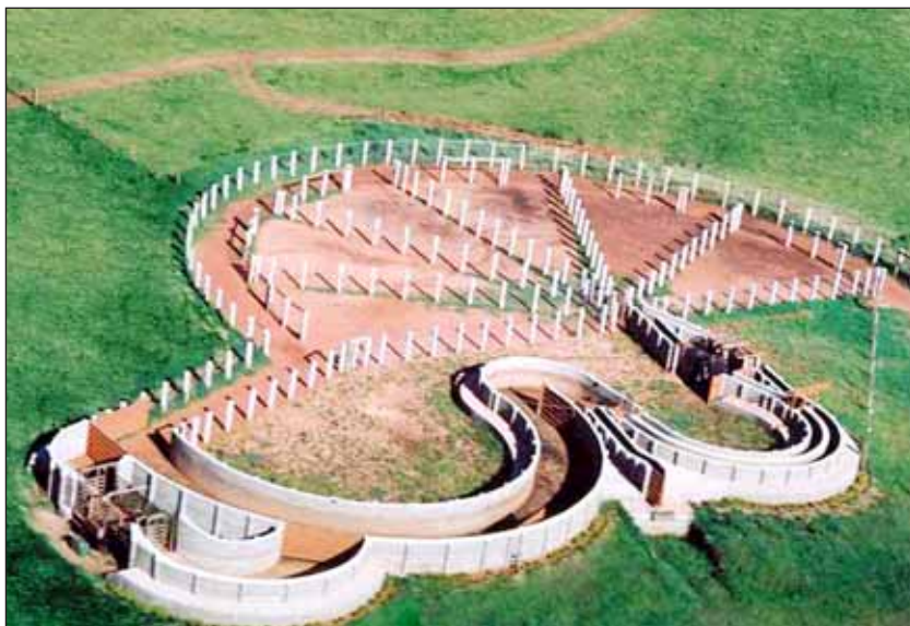
Curved races facilitate the movement of cattle through the cattle handling facility. Photo: Temple Grandin ( www.grandin.com )
