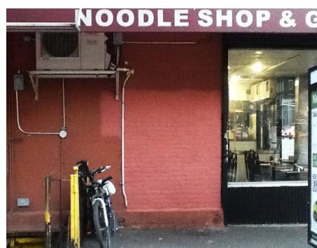
The wall, before and after, above.
