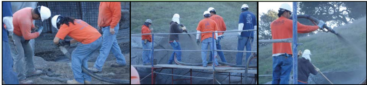
Unplugging the shotcrete hose
