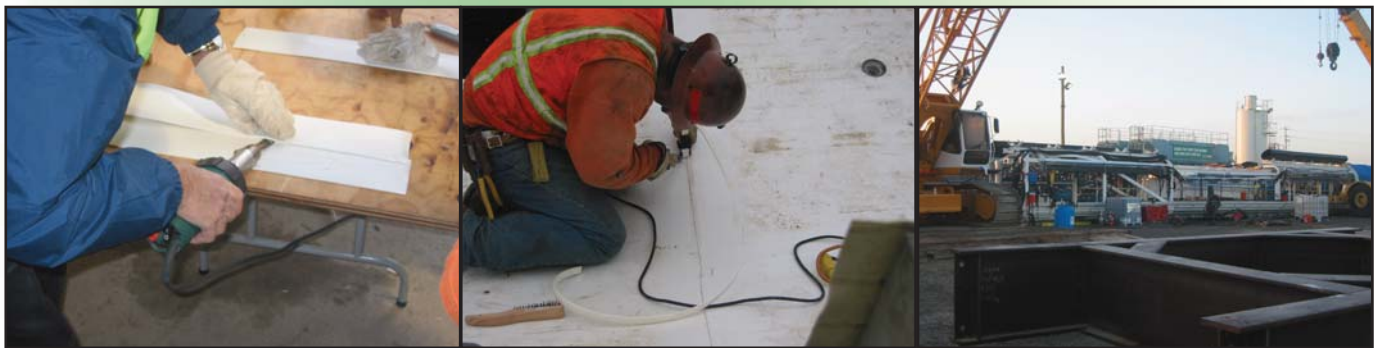
“Welding” seams with T-Lock compound in classroom and hands-on.
