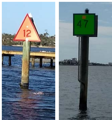
Figure 2.4. Red triangular and green square dayboards. (Note the yellow square and light at the top of the post on #47. [Photos by the author.]
