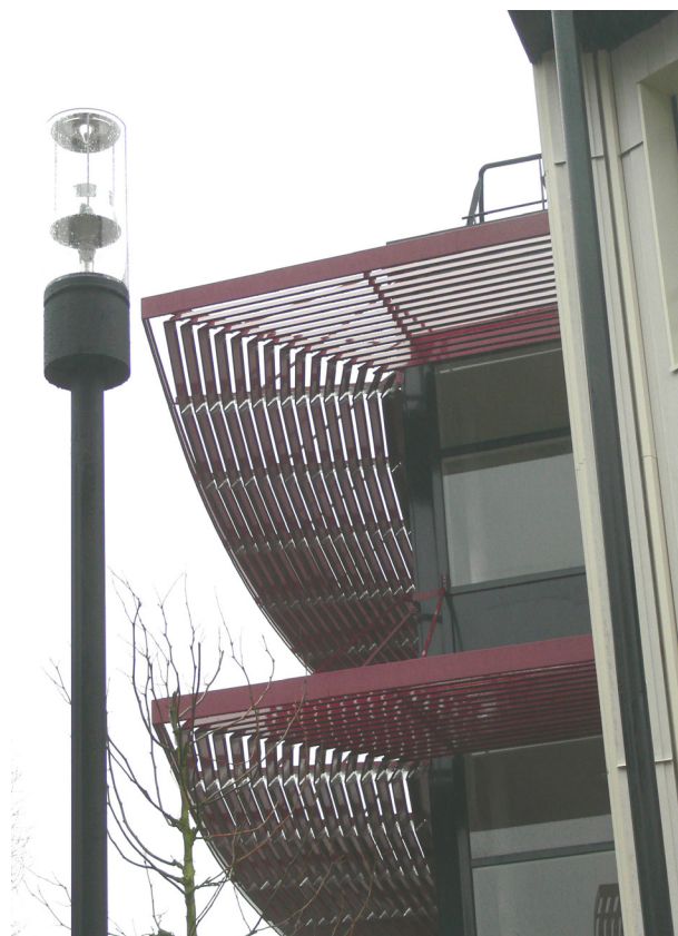
Window overhangs for shading
