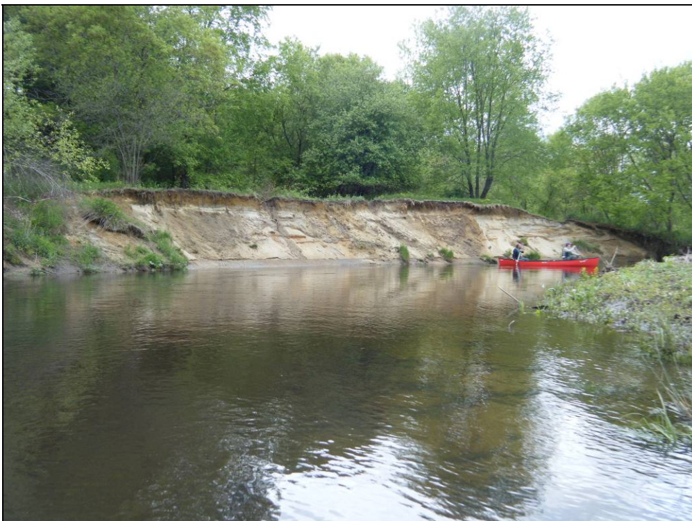
Example of bank conditions with a BEHI rating of extreme
