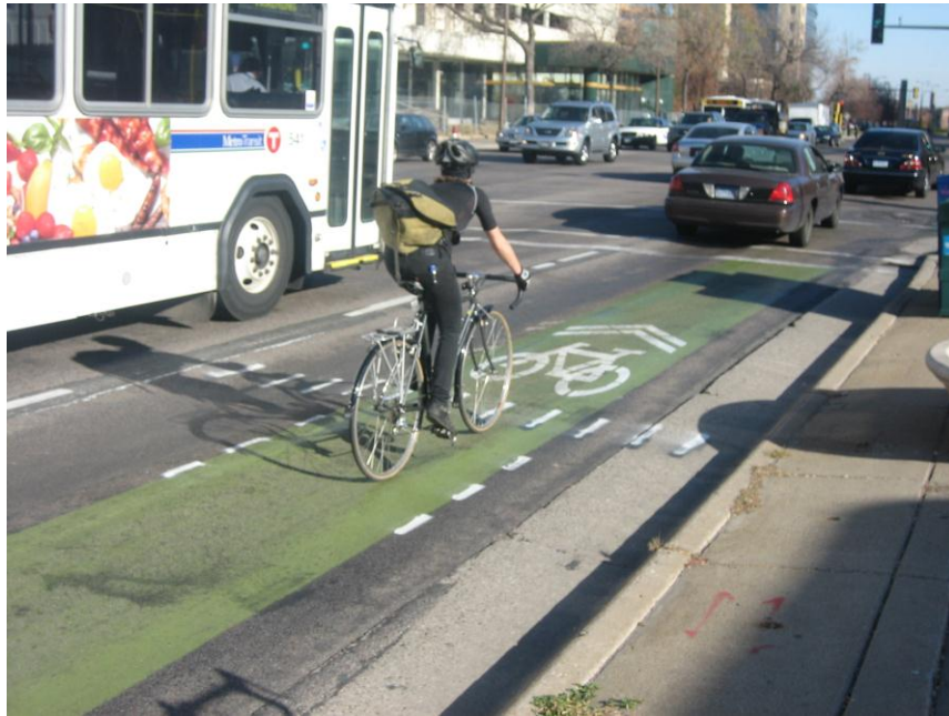
Figure 1.9 – Hatch marks were used to measure lane position of bicyclists and motor vehicles
