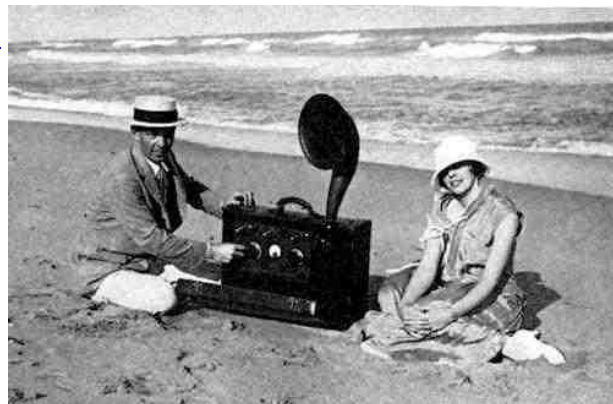
Say it with flowers a radio. In 1923, as a wedding present (and publicity photo) at Palm Beach, Florida, Edwin presented his bride with the world's first portable superheterodyne receiver, which he built.
