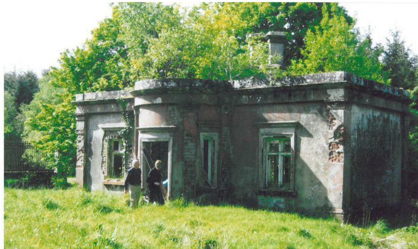
Figures 2.17 & 2.18 Below are before and after images of the Triumphal Arch Lodge, Colebrook, Co. Fermanagh recently restored by the Irish Landmark Trust
