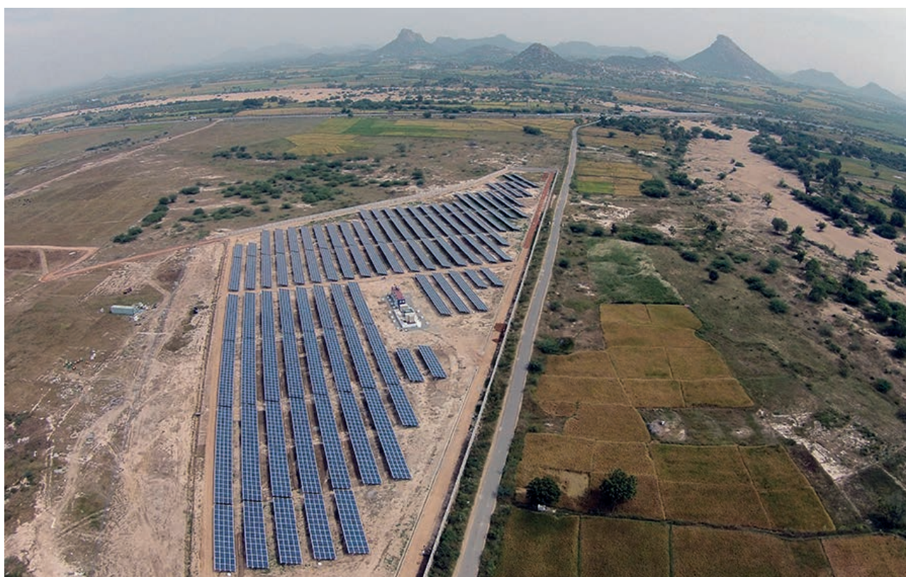
Figure 5: Aerial view of solar photovoltaic plant in Andhra Pradesh, India
