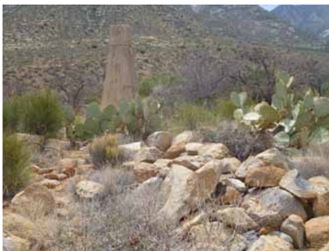
Mt. Graham tramway tower. Photo by Jim Vaaler.
