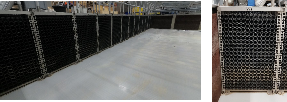
Figure 2-3: Passive absorber elements
