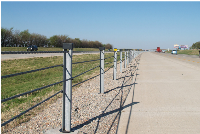
Figure 6-4. Brifen Wire Rope Safety Fence
