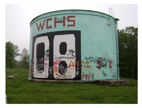
The 300,000-gallon Main Water Tank is a welded-steel, painted tank which fills from the high service pumps at the WTP. The tank needs painted and secured with a perimeter fence.
