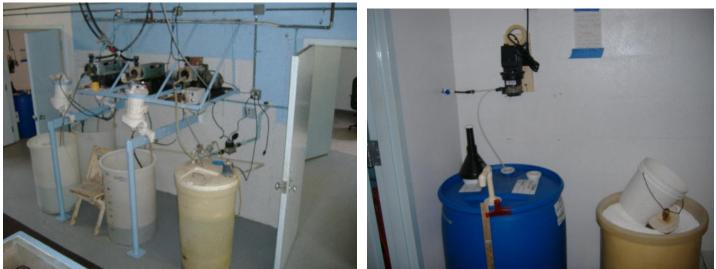
The two photos above show additional chemical feeders which add fluoride and soda ash (left photo) and the primary coagulant, DelPAC 2020 (right photo).
