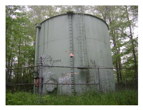
The Secondary Water Tank is primarily used for fire protection. The paint condition of the welded-steel tank was judged to be in generally good condition, with some oxidation of the paint and some graffiti on it. The security fencing is in poor condition around the tank site and needs to be either repaired or replaced. There is no telemetry on this tank.
