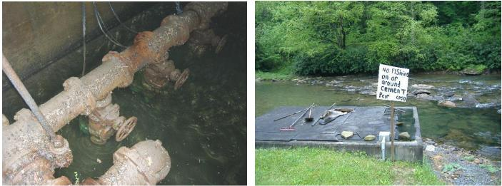
The left photo above is looking into the raw water wet well, which contains three 5 HP Crane Deming raw water pumps, each rated at 330 gpm. Normally two pumps operate together to transfer ~450 to 500 gpm to the water treatment facility. The photo at right shows the intake structure which is partially covered to conserve heat during the winter months.
