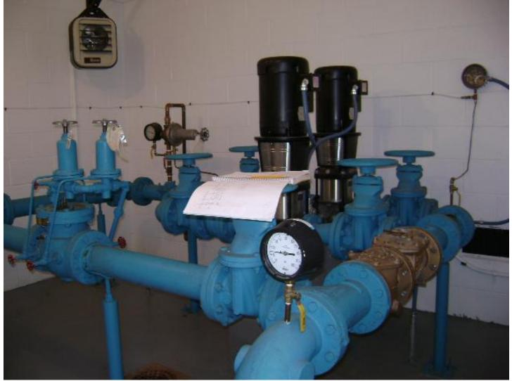
The Osceola BPS is housed inside a locked brick building. The BPS contains two Grundfos Pumps, rated at 150 gpm @ 115.1' TDH. According to the daily log at the BPS, Pump #1 had operated 36 hours between April 30 and May 28, 2008 (inclusive), and Pump #2 had operated 36 hours during the same period. Thus, it can be
