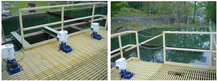
After being dosed with the primary coagulant, DelPAC 2020, and chlorine, the water enters a 3-stage flocculation chamber. Each of the three drive units in the upper left photo mixes the water at a progressively slower rate, to form a floc which then settles out in the sedimentation basin. The 3-stage flocculator holds about 17,500 gallons, thus providing a theoretical detention time of about 38.8 minutes (i.e., assuming a production
