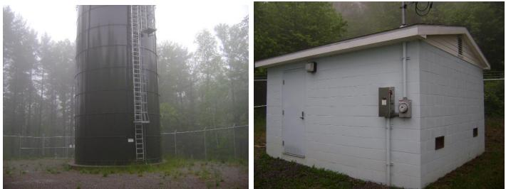
The Osceola Tank (left photo) is filled from the ABC Tank through the Osceola BPS (right photo). The tank is telemetered to the WTP. The tank operating levels are between 48' and 53'. The Osceola tank holds ~125,000 gallons. The Osceola BPS is located beside the ABC Tank, locked inside the same perimeter fence.
