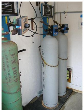
There are two sides to the chlorine/SO<sub>2</sub> building. The photo above is looking into the right side of the building which houses the 150-lb chlorine gas and SO<sub>2</sub> gas cylinders. The cylinders in use are chained to platform scales. The room is equipped with a vent fan, light and room heater.
