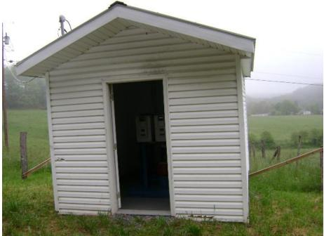
The Main Water BPS is housed in a secure building. According to the daily log between April 2 and May 28, 2008, 162,000 gallons were pumped or an average of 2,893 gpd.
