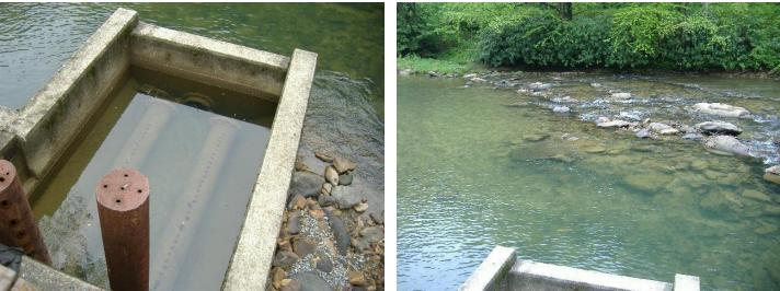
The photo above, left, shows the raw water intake structure on the Maumee River. Flow from the river enters the concrete box and then passes through the pipe perforations into the raw water wet well. The right photo shows the makeshift impoundment on the river, made with river rocks, which helps to pool river water at the intake.
