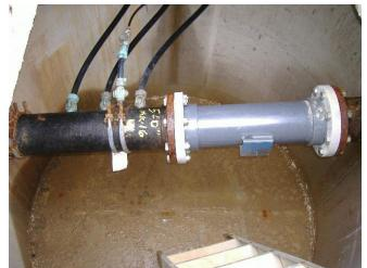
Prefed chemicals are injected into the raw water line, inside a below-grade concrete vault, which contains an inline static mixer. During the recent survey DelPAC 2020 and chlorine gas were being prefed at this location. KMnO4 was also being prefed, but it was being added at the first stage flocculation unit.
