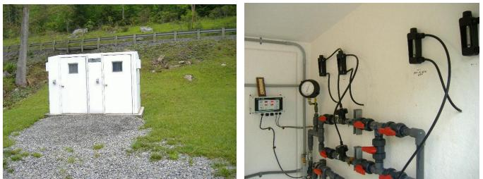
The gas chlorination building is located across the driveway from the WTP. This building also houses an SO<sub>2</sub> feed system which is used to dechlorinate filter backwash water. During the recent survey chlorine gas was being pre-fed at about 5 lbs/24 hours (0.92 ppm) and postfed at about 7 lbs/24 hours (1.28 ppm).
