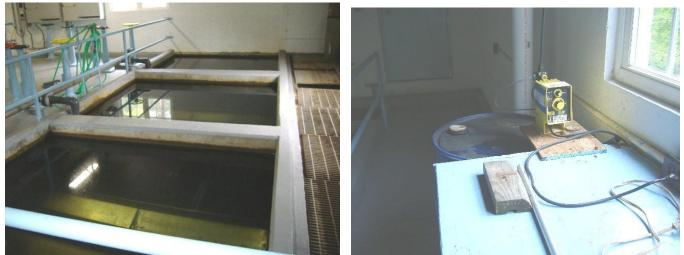
Three 60 ft<sup>2</sup> filters (left photo above) provide final filtration of the water to comply with the requirements of the LT1ESWTR which requires a combined filter effluent of  $\leq 0.3$  NTU at least 95% of the time. The right photo above shows the KMnO<sub>4</sub> feeder which is located in the filtration room.
