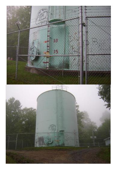
The ABC tank is filled by the high service pumps at the WTP. The inside of the tank was cleaned and inspected in 2005. The tank is telemetered to the WTP.
