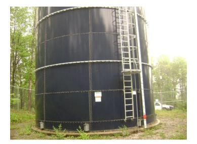
The Business Park tank is also filled by the high service pumps at the WTP. This tank is an Aquastore, glasslined, bolted-steel tank. The 108,000-gallon tank is 29 feet tall. Key tank facilities are secured with a perimeter chain link fence which was installed in 2004.
