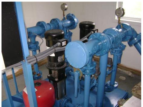
Dual Grundfos Vertical Pumps, series C, rated at 55gpm @ 245' TDH, run continuously, and draws from the Main Water Tank to maintain a line pressure of 75-80 psi to system customers.
