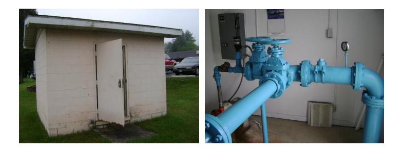
The Secondary Water BPS is housed inside a locked brick building (left photo). The pump is regulated on a timer and runs about 3-4 hours a day. The telemetry is broken. The Secondary Water BPS pumps water to the Secondary Water Tank.
