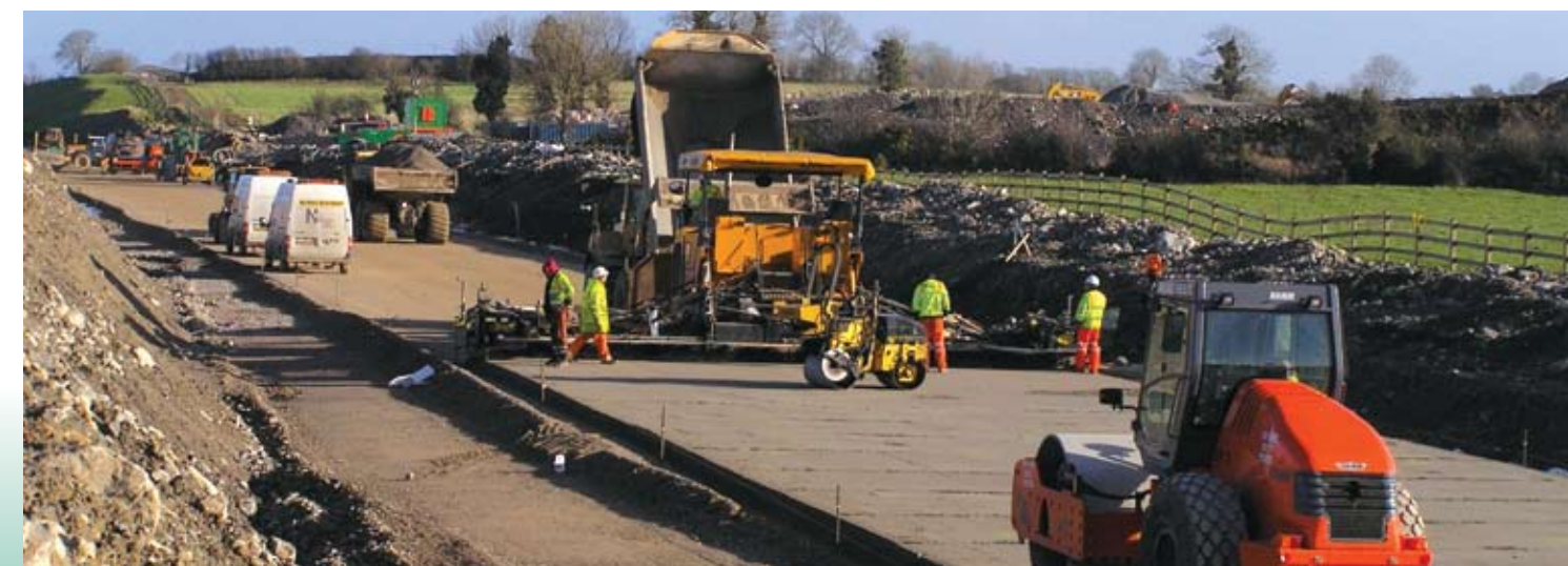
ROAD CONSTRUCTION WORKS
