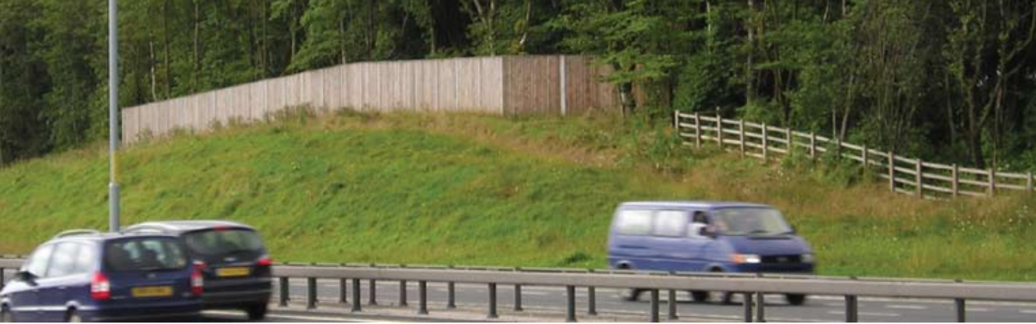
EXAMPLE OF TIMBER NOISE BARRIER
