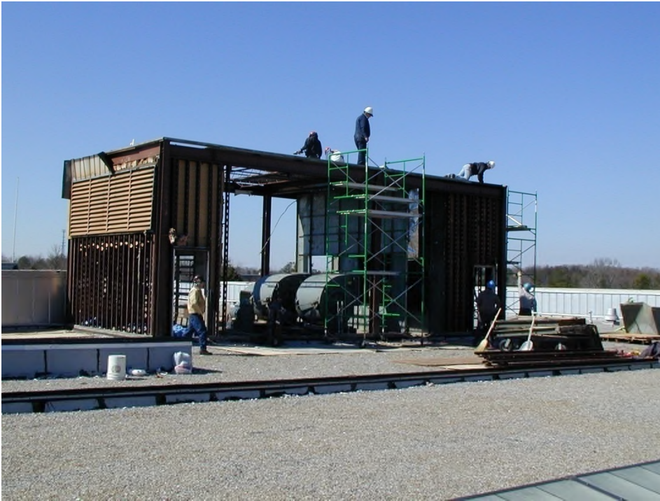
Existing roof built unit
