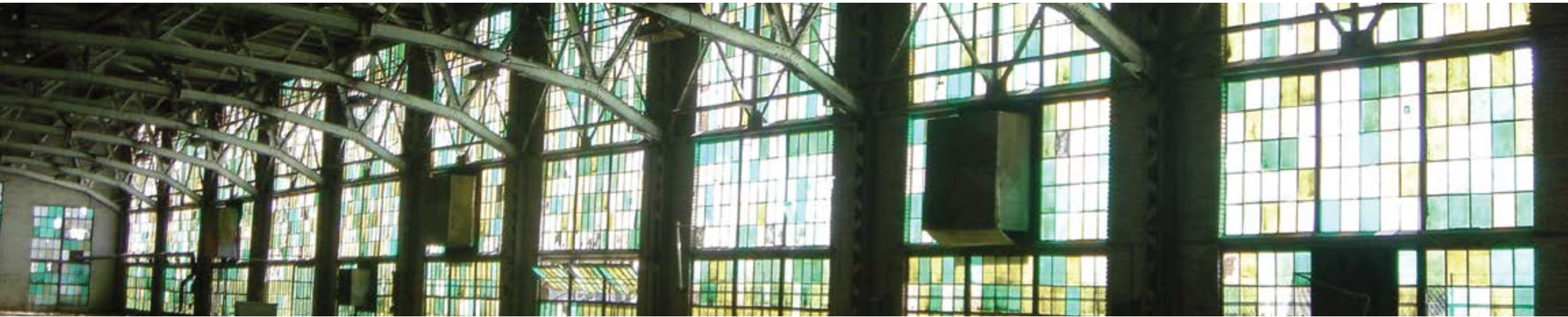
Former Albuquerque Rail Yards Site (Photo courtesy of Bill Tondreau)
