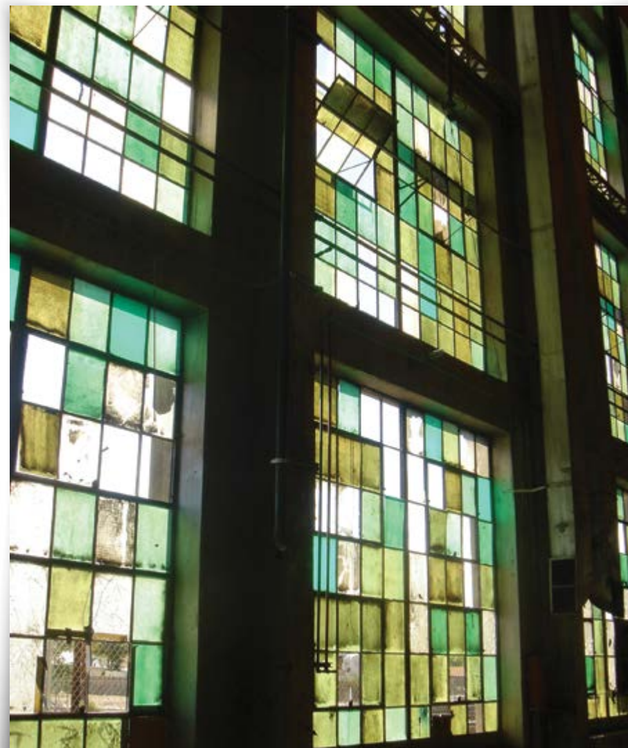
Former Albuquerque Rail Yards Site (Photo courtesy of Bill Tondreau)
