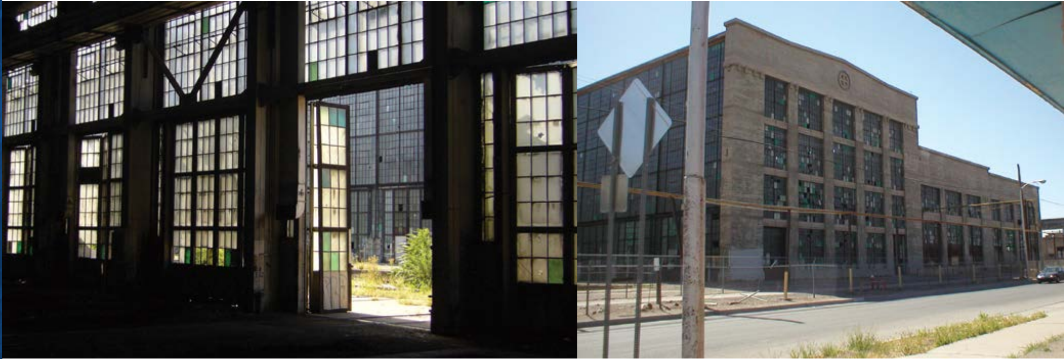
Former Albuquerque Rail Yards Site (Photo courtesy of Bill Tondreau)
