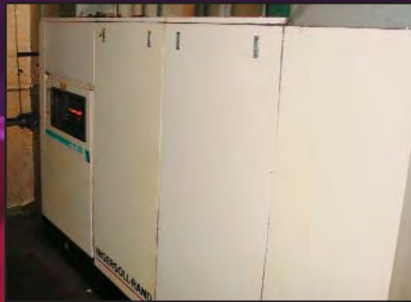
VIEW OF INGERSOLL-RAND ROTARY SCREW AIR COMPRESSORS
