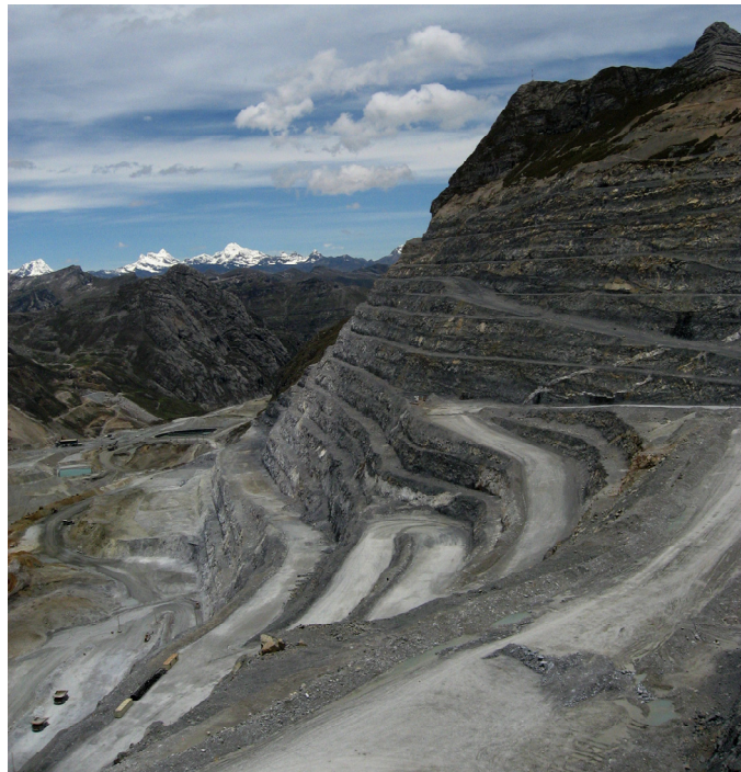
Figure 9 - Geotechnical benches on an open pit slope (photograph courtesy of Compañía Minera Antamina S.A.)
