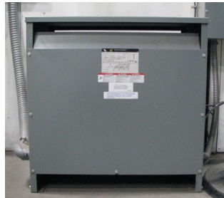
Figure 1 Small Dry-Type Transformer Shermco Industries, Inc.
