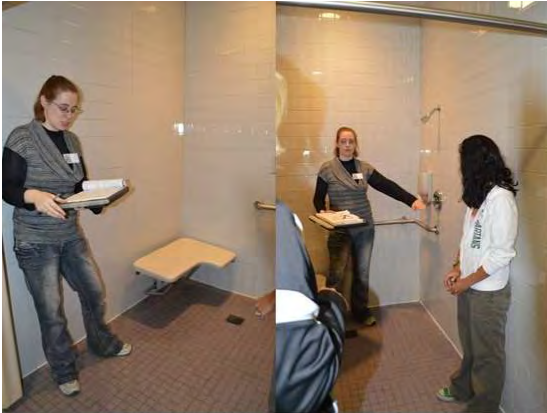
Figure 21: Accessible shower compartment. Photo courtesy Marylu Dykstra, Disability Advocates of Kent County.
