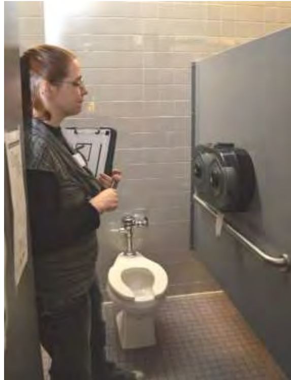
Figure 19: Ambulatory Accessible Toilet Stall. Photo courtesy Marylu Dykstra, Disability Advocates of Kent County.
