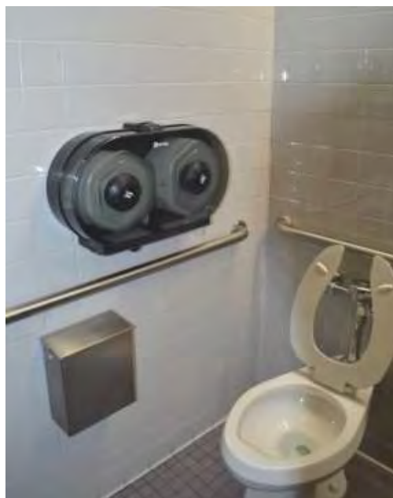
Figure 20: Wheelchair accessible toilet stall. Photo courtesy Marylu Dykstra, Disability Advocates of Kent County.
