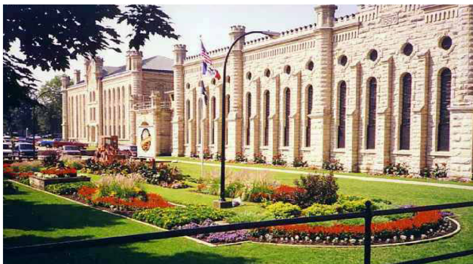
Construction of the stately Anamosa State Penitentiary began in 1874 using stone from a local quarry. Cells were four feet, 6 inches wide, seven feet six inches in height, and eight feet in length. It was almost ten years later that electric lights were first used.
