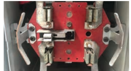
Figure 11 – Replacement socket for gen 2 and gen 2.5 Uni-Pak devices: MMSCK1
