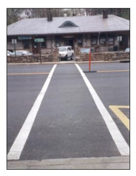
Picture 3.1-1: Crosswalk leading across multi-lane road to the train station – unsafe due to long distance, high speeds of traffic and no refuge for pedestrians. Bernardsville, NJ.
