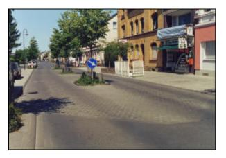
Picture 3.2-1: Cobblestone surface texture and tree planted islands to reduce motor vehicle speeds. Germany.
