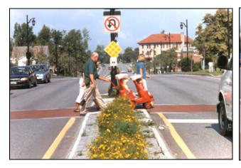
Picture 3.3-1: Insufficient width of median refuge. Burlington, VT.
