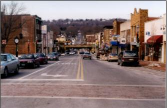
Picture 4-8: Main Street (after) with one lane in each direction and center turning lanes, paved crosswalks and widened sidewalks. South Orange, NJ.
