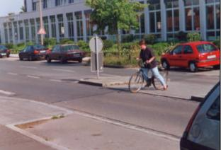
Picture 3.3-2: Sufficient width of median refuge. Germany.
