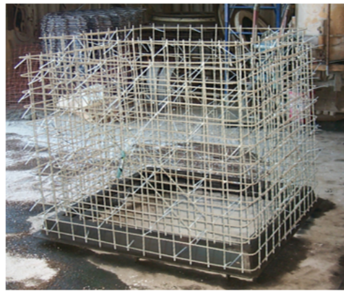
Fig. 2—A complete GFRP cage before concrete casting
