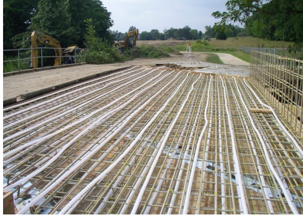
Fig. 4—Southview Bridge deck top-GFRP layer and CFRP tendons
