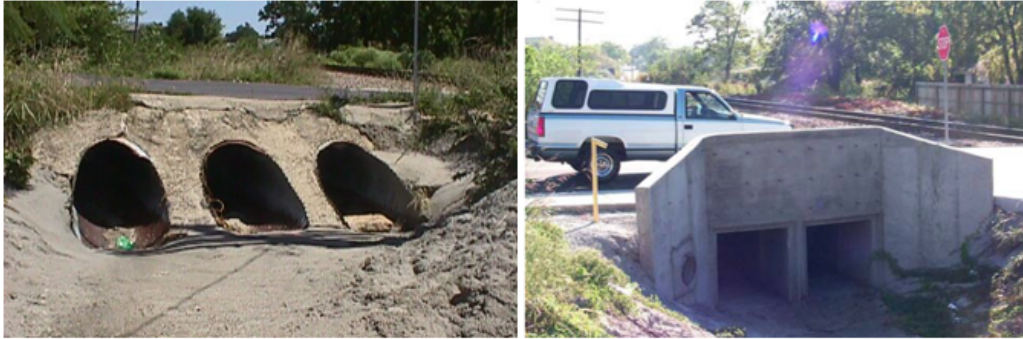
Fig. 1—Old (left) and new (right) Walker Bridge
