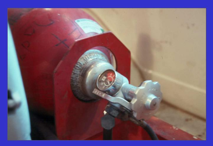
Check nitrogen tank gauges to ensure they are not discharged or below minimum pressure
