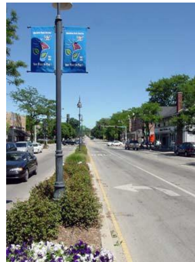
Figure I-3: Traffic Calming: Landscaped Portion of a Pedestrian Refuge Median in Downtown Glenview, Illinois
