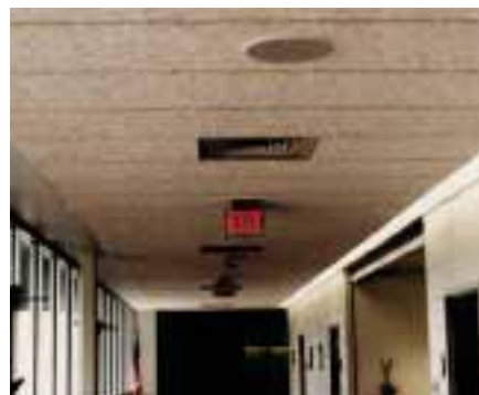
▲ Royal Middle School (Pattison, TX) Full-Span Corridor Panels
