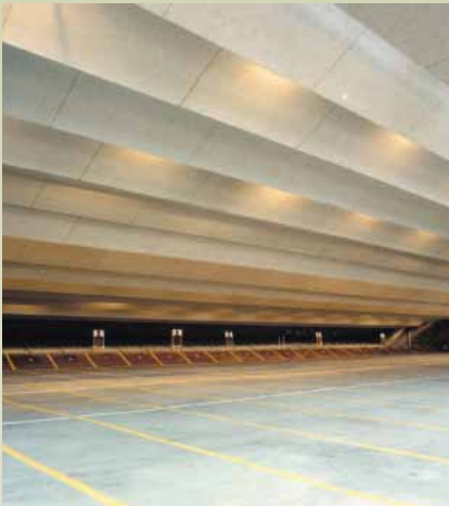
▲ Police Department Firing Range (Los Angeles, CA) Tectum Hanging Baffles
