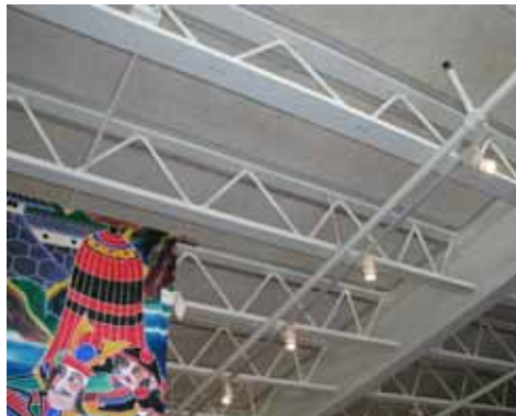
◀ Beacon Building (Culver City, CA) Direct-Attached Ceiling Panels
