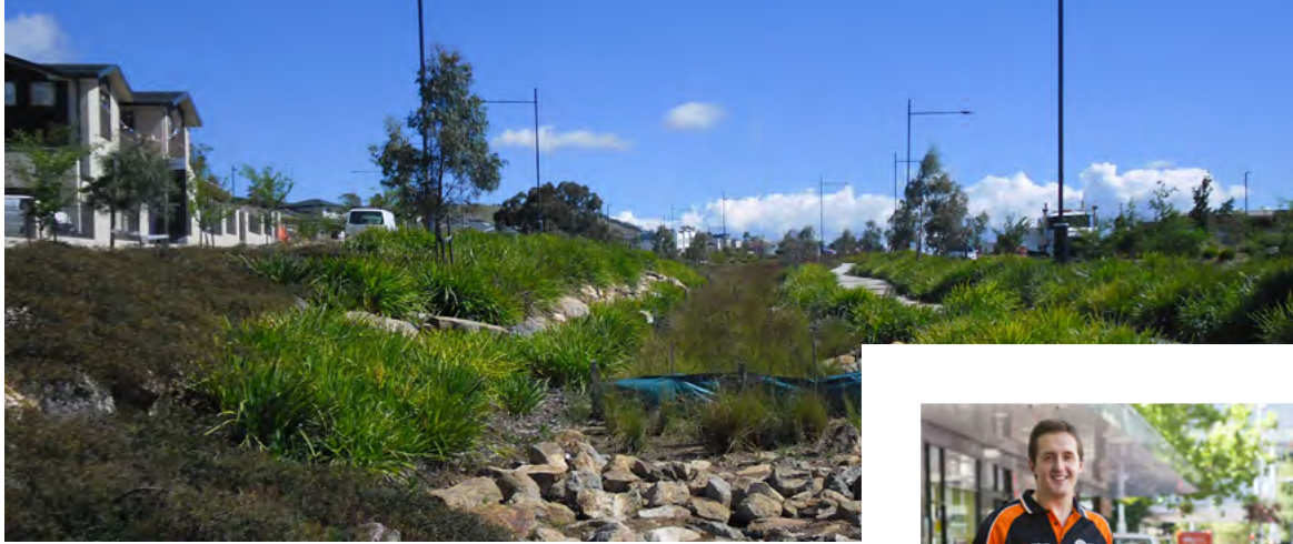
WSUD landscaped swale located in Plumsoll Ave, Casey
