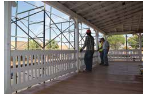
Crews restore the second floor porch of the Armijo House.
