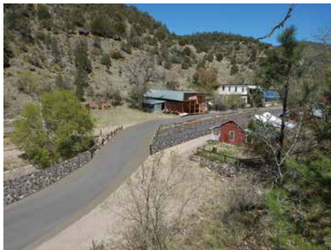
Parametrix's rendering of the lower entrance to town shows how the new road and associated improvements will look. Historic reviews for this project were fast-tracked by HPD.
