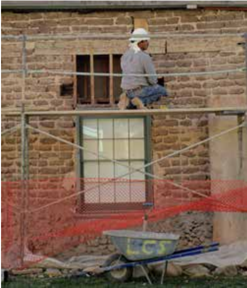
Empty space above downsized windows is repaired by a worker installing a lintel. Cobblestones, firebricks and cement blocks were found indicating repairs from different eras. The skeleton key found hanging from a square-headed nail beneath old plaster.
