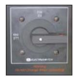
Three Position Padlockable Voltage Selector Switch
