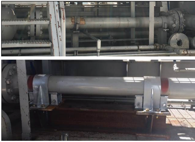
Figure 14. Discharge Pipe Supports Replacement
