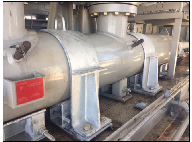
Figure 13. Discharge Bottle Support Replacement
