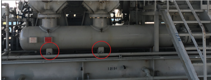
Figure 11. Discharge Pulsation Bottle Supports As Initially Installed
