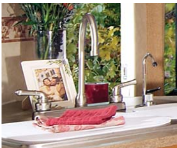
Residential galley faucet, water filter with spout & sink covers
