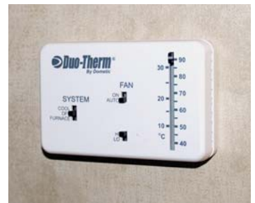
13.5 BTU air conditioner with wall thermostat
