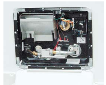
Gas/electric water heater with DSI
