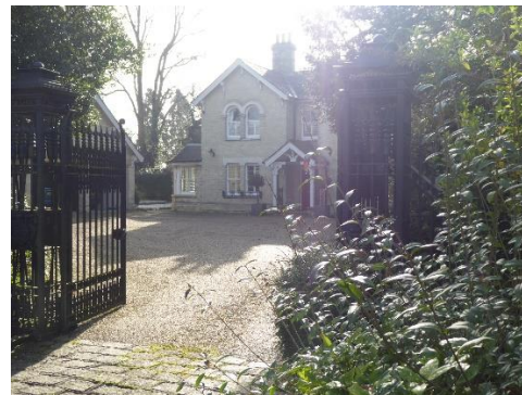
Left: distinctive glazing patterns at 32 and 28 Mingle Lane
