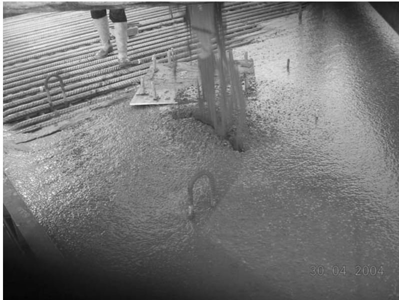
Figure 6-42 Application of self-compacting concrete for in situ piles
