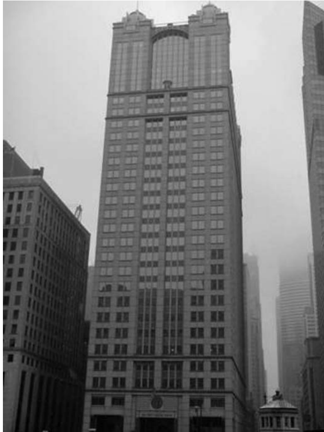
Figure 1-5 The 225 West Whacker Drive building in Chicago, Illinois, USA (Photo provided by Xiaojian Gao)
