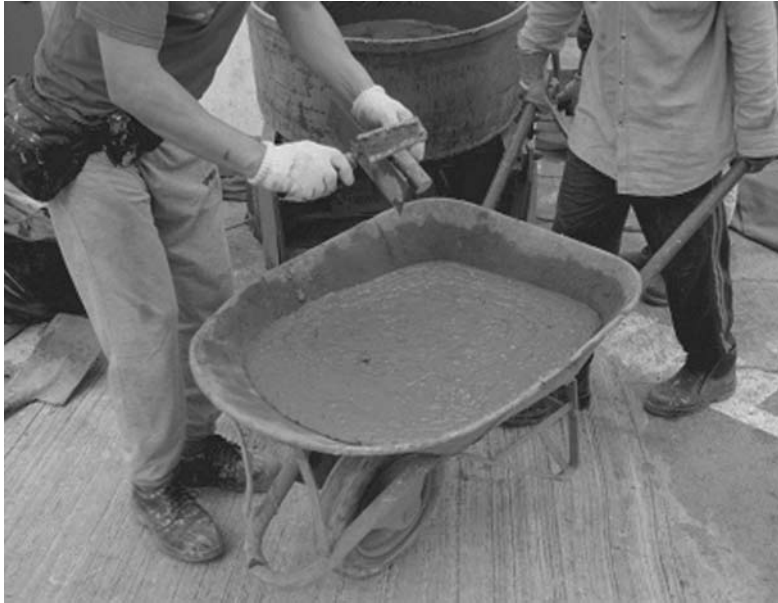
Figure 3-19 Wheelbarrow used on construction site
