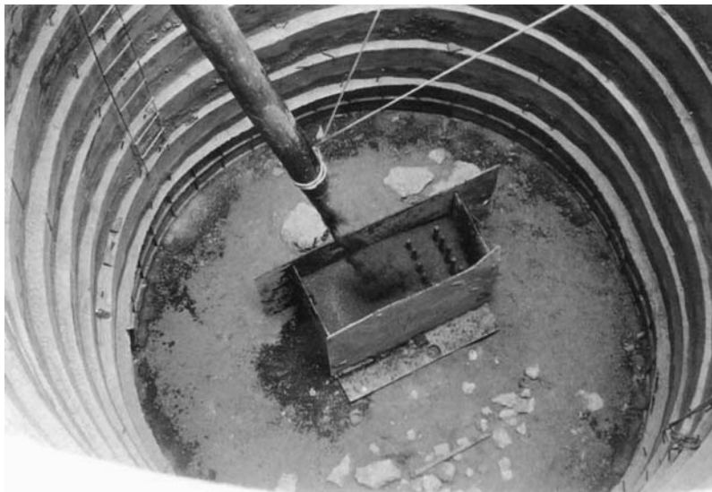
Figure 3-21 Drop chute-guided concrete fall
