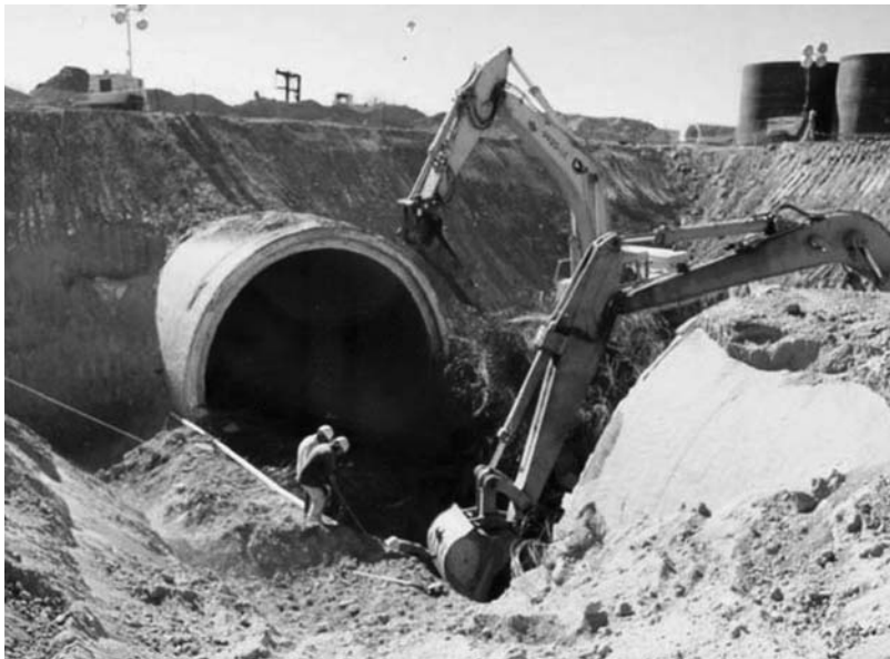
Figure 1-11 Pipeline under construction (Photo courtesy of Exponent, http://www.exponent.com/corrosion_analysis_of_pre_stressed_concrete_pipeline/ )
