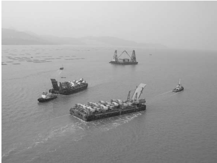
Figure 3-14 Delivery of concrete to an ocean construction site using a ferry (photo provided by Ove Arup, HK)
