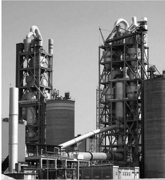
Figure 2-8 A production line of 10,000 metric tons per day (Hai Luo Cement Company, China)
