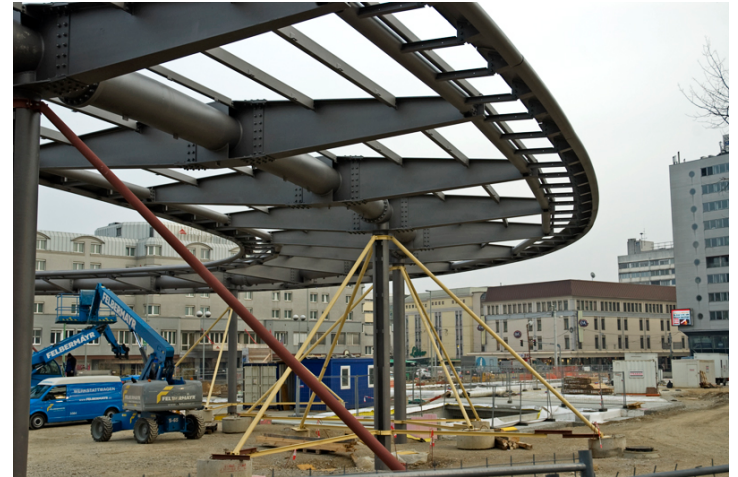
Construction site in front of the Central Station, Europaplatz, Graz, Austria
