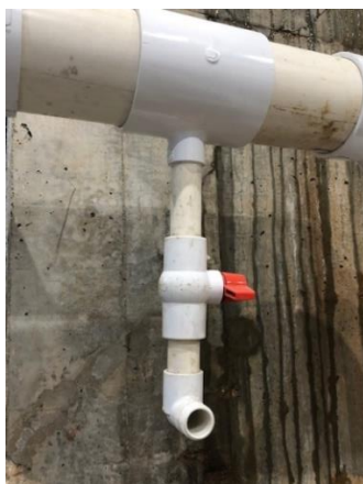
Figure 6 Photograph of Background Sampling Port
