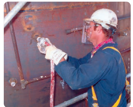
Kaowool pumpable being pumped to repair hot spot
