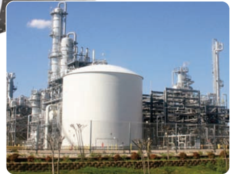
Above ground storage tank
